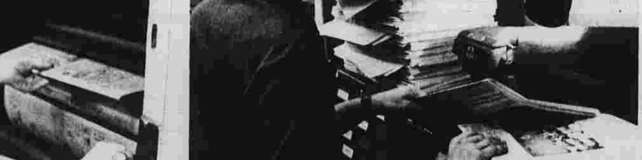
After the newspaper page is assembled in the composing room, it goes through a process in which the page is photographed and converted to a printing plate. Here, pressman Roger Schuetz fixes a printing plate on The Herald's offset press.
